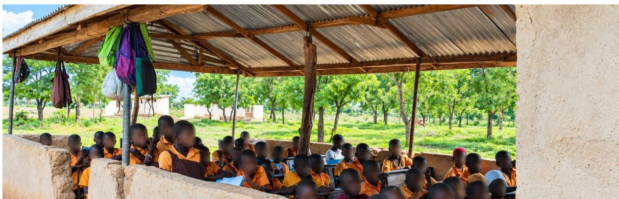
Ongoing teaching and learning in a dilapidated Tuyini D/A Primary in the Sung Circuit
